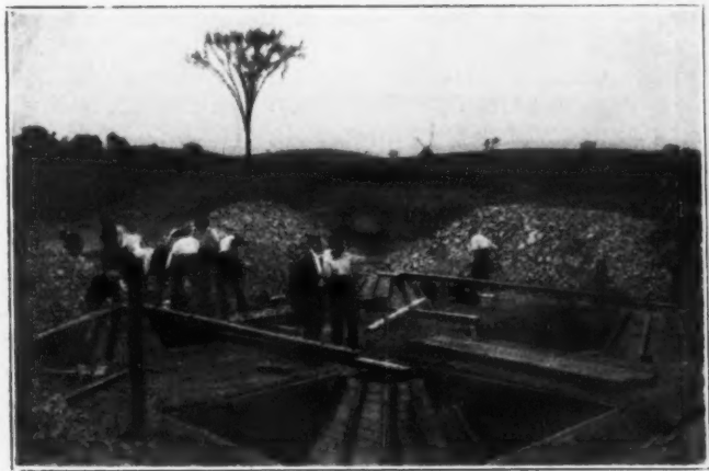
FIG. 22—CONCRETING FOOTINGS FOR SPECIAL NEW YORK CENTRAL CROSSING
